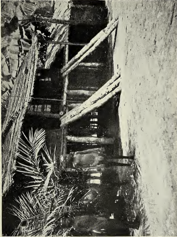
A FOMA COTTAGE ON LEGS. Leaves of primer stuck in the walls.
